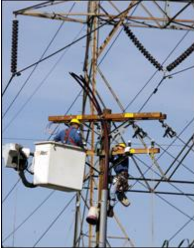
Workers repair damaged lines
